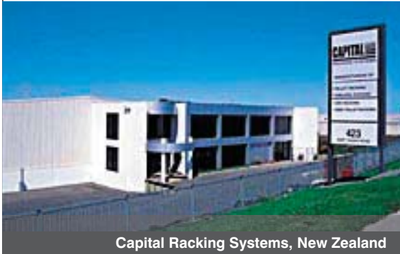
Capital Racking Systems, New Zealand
